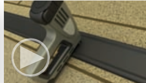
Tack with staple gun or nails, install metal roof on top
