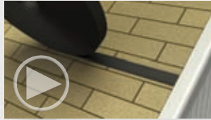
Unroll across existing shingle roof
